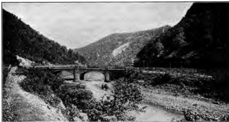
Old National Bridge, Cumberland
